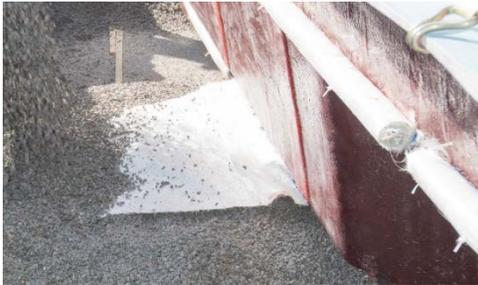
**STEP 4: FINISHING STEPS:** Continuing backfill as normal. The top of the Geo-Hydro Valve is finished off with the Waterway Skimmer Lid and Collar. An extension collar may be needed depending on the height of the coping.
