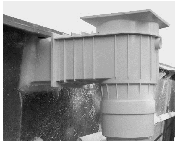
11: Generously apply silicone to the backside of the skimmer as shown.
