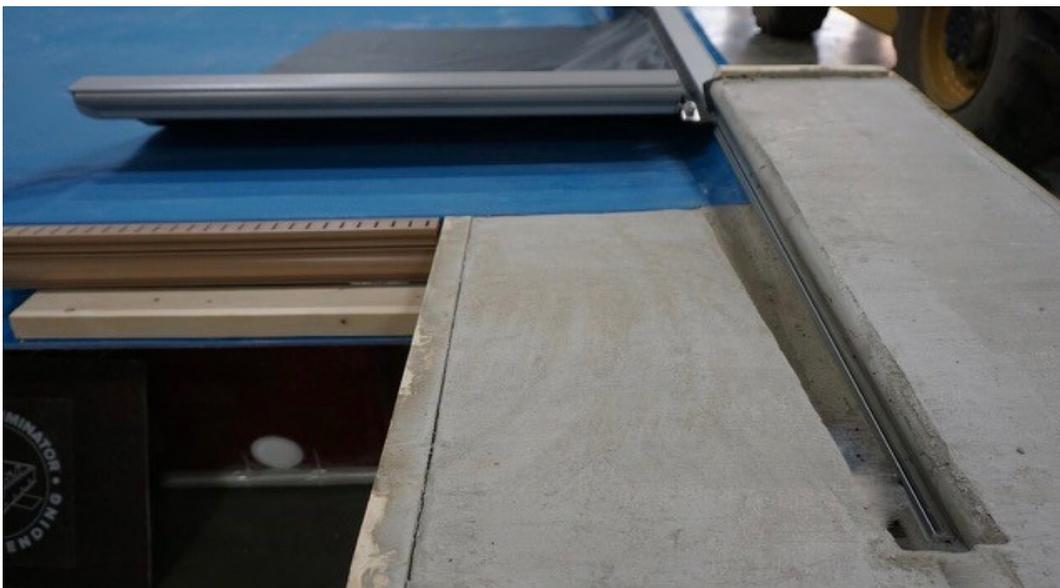
*Concrete pour that allows for automatic pool cover to reach top of slope.*
