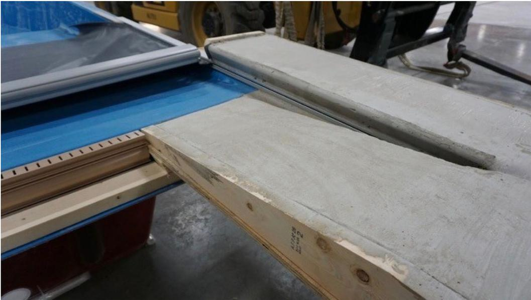
*Concrete pour that allows for automatic pool cover to reach top of slope.*
