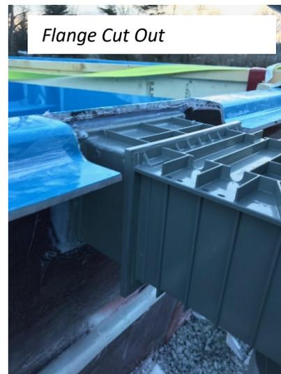
**\*\* Critical\*\*.** Your skimmer height directly effects the water level on your beach entry. For every inch of water level, you will create 9" of 'dry' area or exposed fiberglass on the beach entry. To minimize the amount of fiberglass exposed, place the skimmer at the top of the pool wall. See image below. Add Water Features to minimize 'dry' area.
